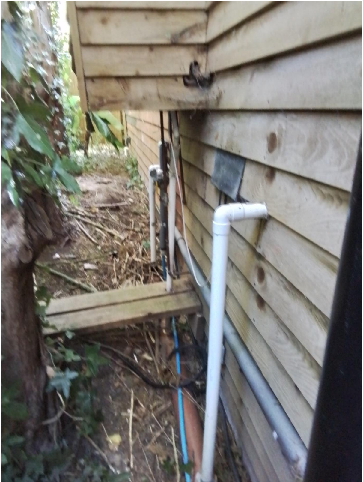
Pipework to the rear west of Treehouse
