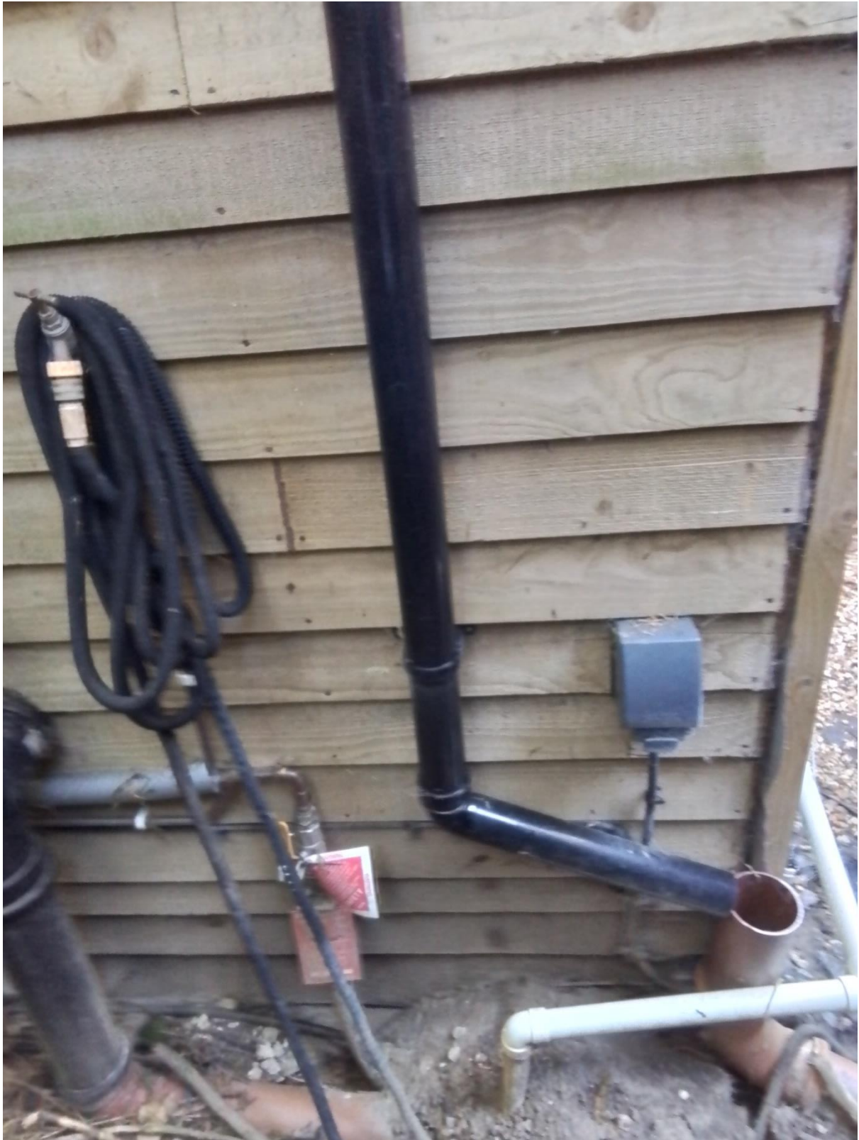
Utilities on SE corner
