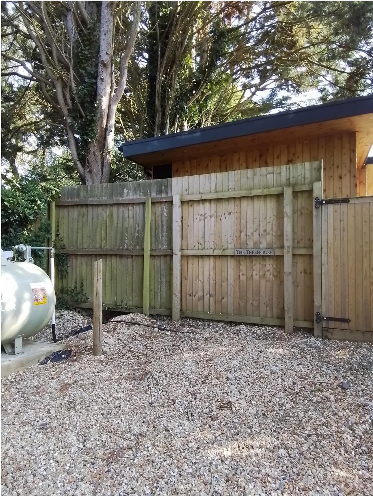
South elevation Tree House from car park
